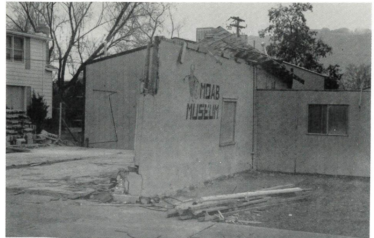
Demolition of the old museum - 1987 - Photo by Kent Dalton
